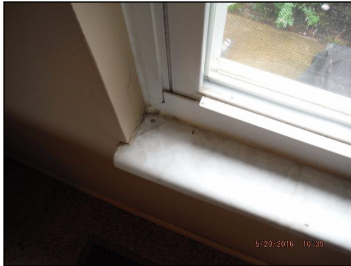
25. Noted what appears to be water staining at...
