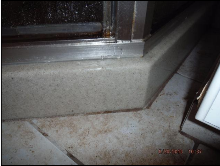
90. Sill and threshold problems
