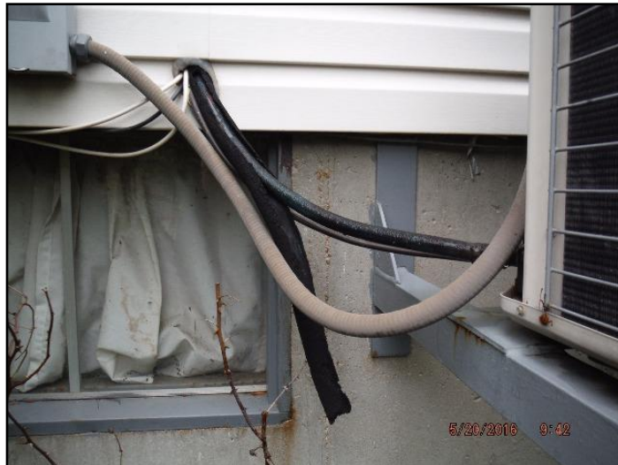
11. Recommend replacement of damaged insulation...
