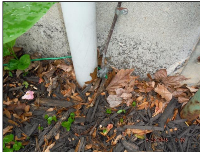
55. Copper - ground rods
