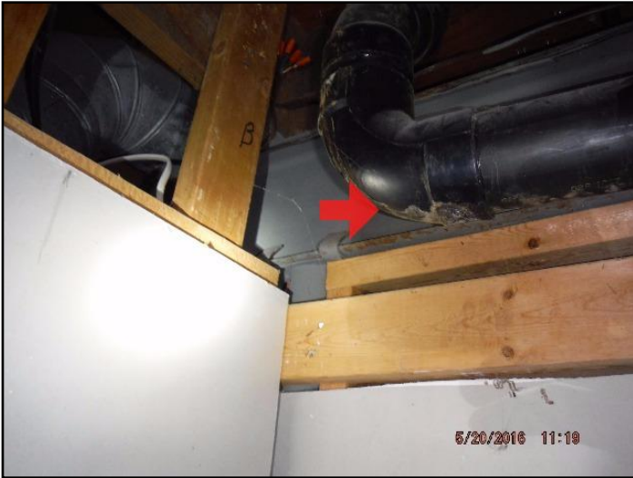
88. Evidence of previous leakage at toilet.
