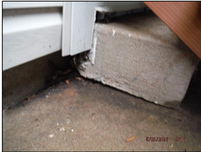
44. Noted settlement of concrete patio slabs at...
