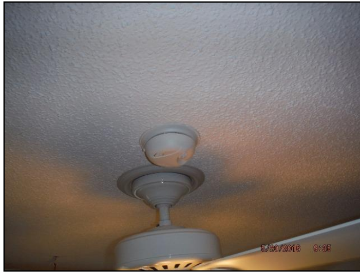
9. Noted improper location of bedroom smoke...
