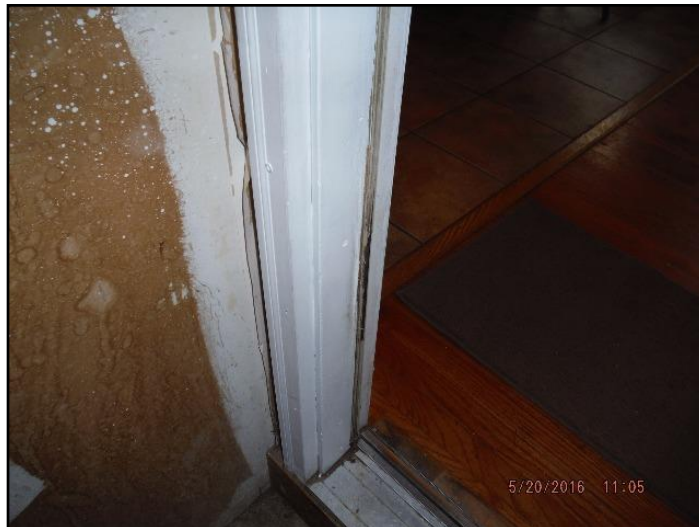
26. Weatherstripping missing or ineffective
