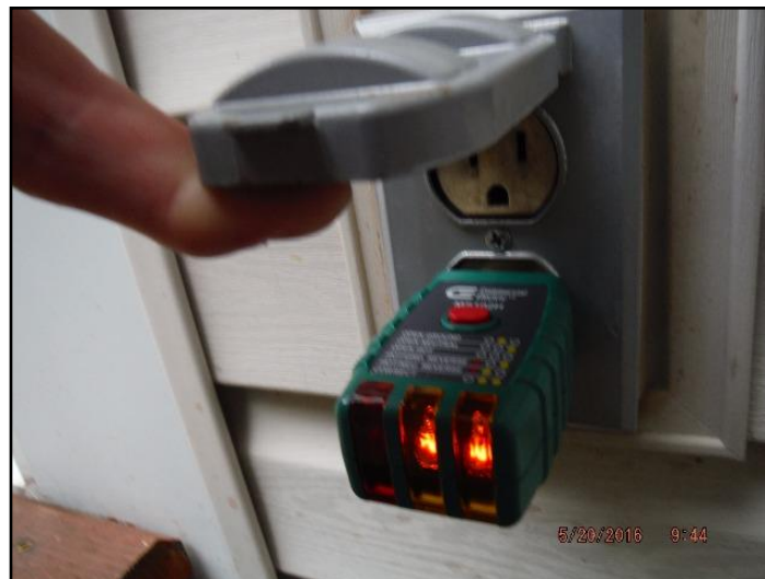
59. No GFCI (Ground Fault Circuit Interrupter)
