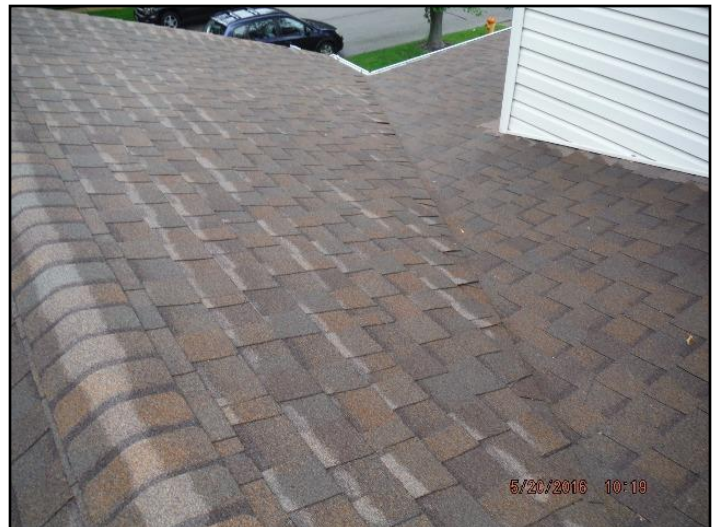
30. Architectural shingles typically have a...
