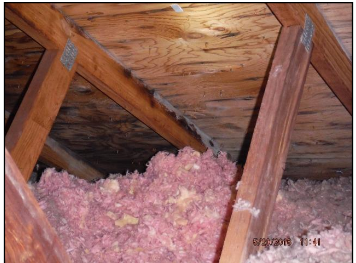
15. Recommend improving attic ventilation
