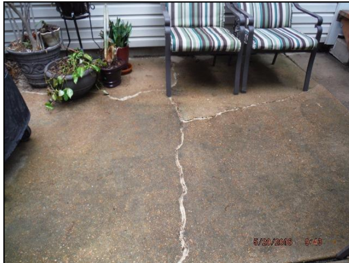
43. Cracking noted in concrete patio. Suspect...
