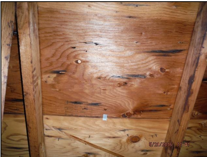
14. Recommend improving attic ventilation
