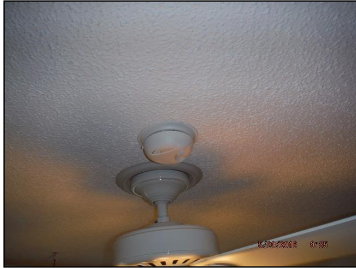
60. Noted improper location of bedroom smoke...
