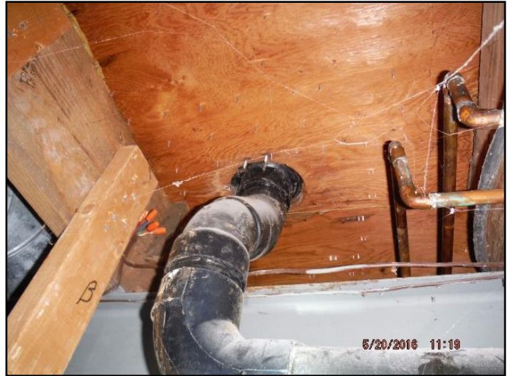
89. Evidence of previous leakage at toilet.
