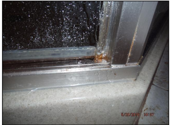
19. Sill and threshold problems
